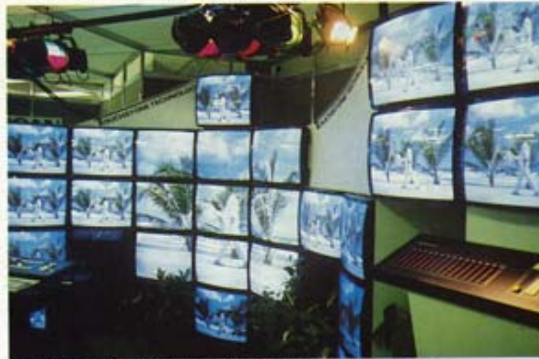
Touchstone Technology - integrated lighting and videowall control.
