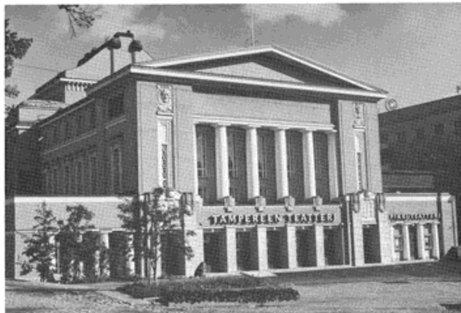
The Tampereen Theatre, originally built in 1913, has just reopened after a major refurbishment.
